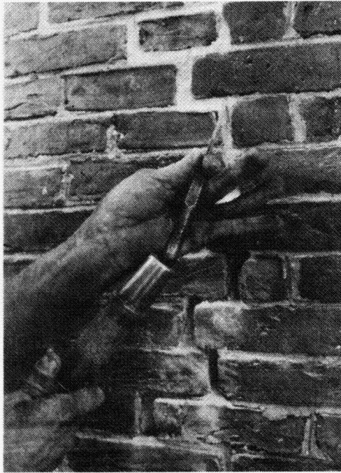
The Trow & Holden pneumatic chisel was developed for sculpture (left), but can also remove old mortar quickly and with little fatigue to the worker. The worker maintains precise control by manipulating the loose-fitting chisel (center), and controlling the pneumatic back-pressure with his other hand. Vertical joints are easily cleaned (right), without harming adjacent brick -- a real problem with grinding equipment.
