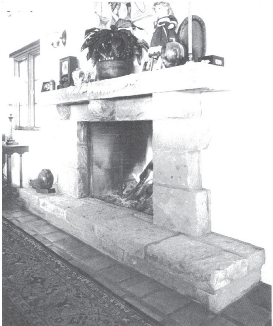
The weighty presence of hand-wrought stonework is entirely in keeping with the study detail in this Spanish Colonial revival style home. Soto used a plywood template to regulate the curvature of the bottoms of the corbels that support the mantel, and he shaped them with a pitching chisel.
